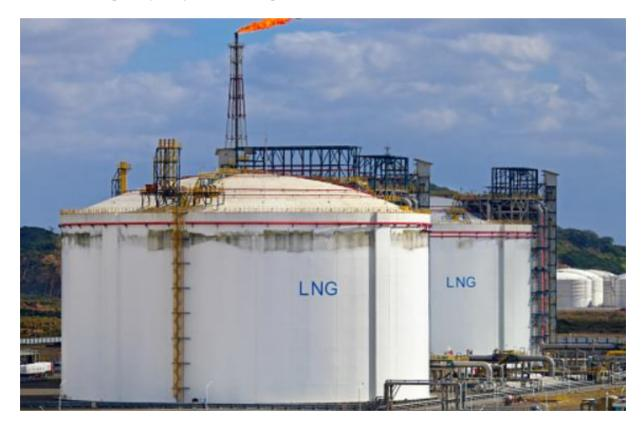
Figure 2: Cryogenic LNG storage (Reuters, 2020)
